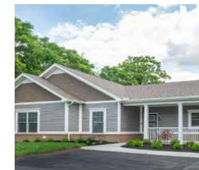
The first Verland Signature Home, located in Monaca
